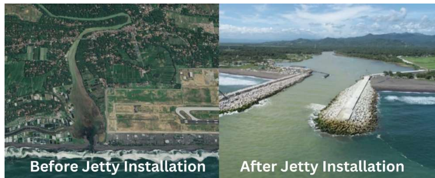
Figure 1. Bogowonto River Estuary Condition, (a) Before Jetty Installation and (b) After Jetty Installation
