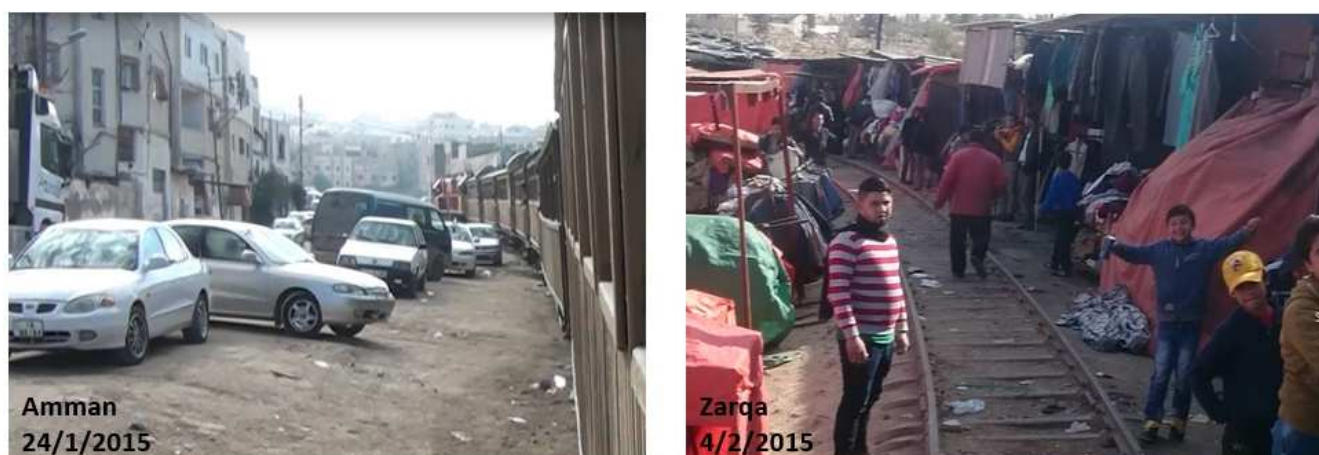
Figure (3-1): Railway Condition in Built-up Areas.
