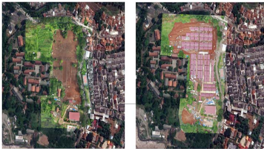
Fig 5. Development of permanent housing Sirnagalih Village [21]
