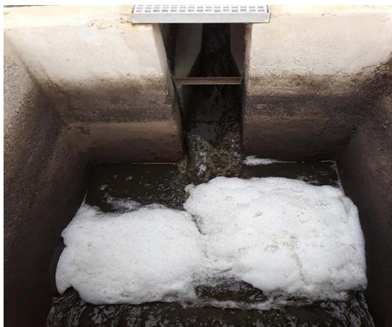
Fig.4: Wastewater after treatment by the WWTP
