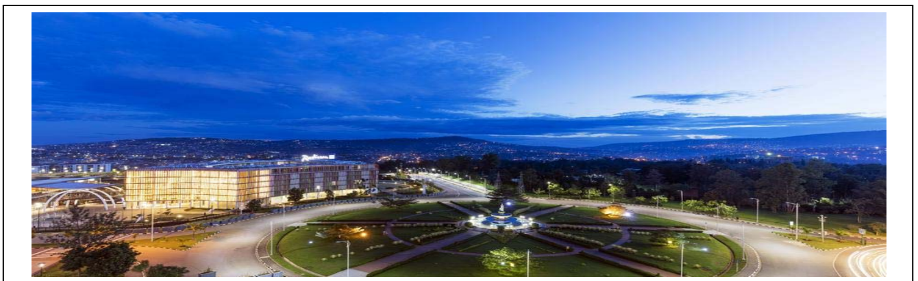
Fig.1.2: Covid-19 and Total Lock down in Rwanda Source: Photo internet
