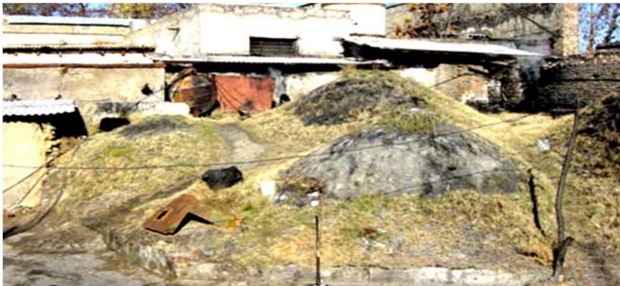
Figure 2. View of the Gungalak underground bathroom.
