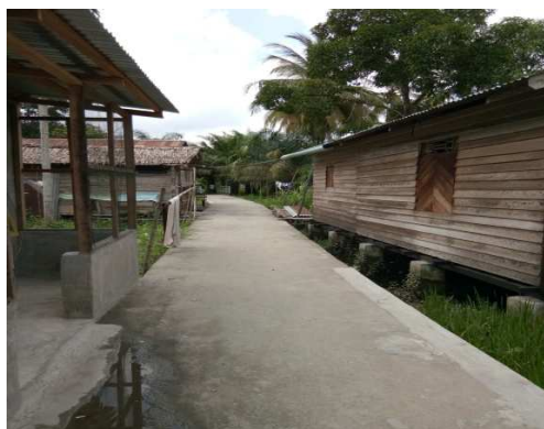
Picture 1: One of the concrete footpath construction in Sirantau
